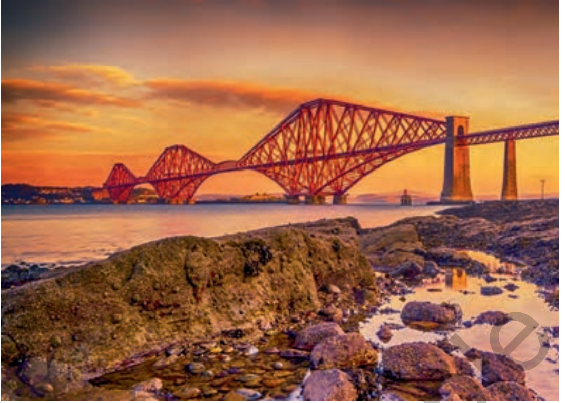
Forth Rail Bridge, Fife
